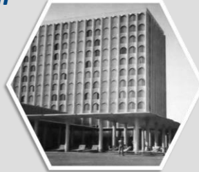
Hotel where I worked
